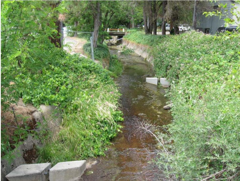
Figure 5. Sidney Gulch (Middle Weaver Creek) cement-lined channel with concrete baffles; coho passage severely limited.
